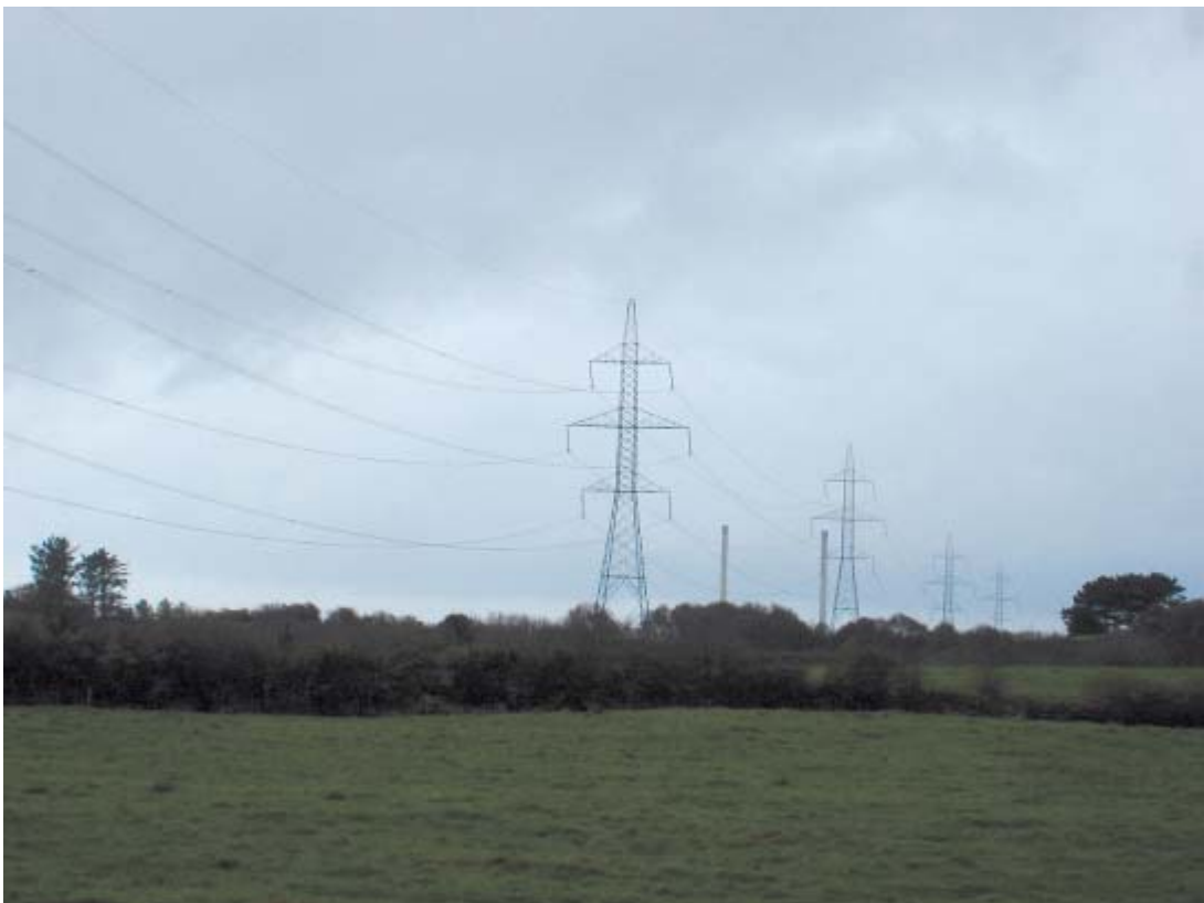
Figure 2.1: Photograph of 400 kV Double Circuit Intermediate Towers
