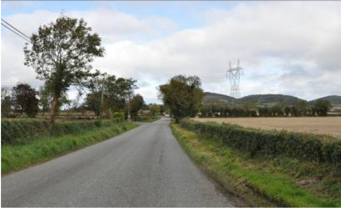
Figure 3.21: R426 Road Looking North Along Route F
