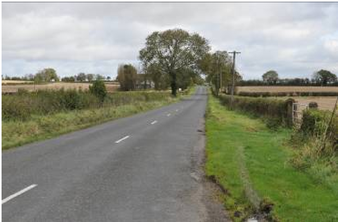
Figure 3.8: R427 Regional Road Looking East
