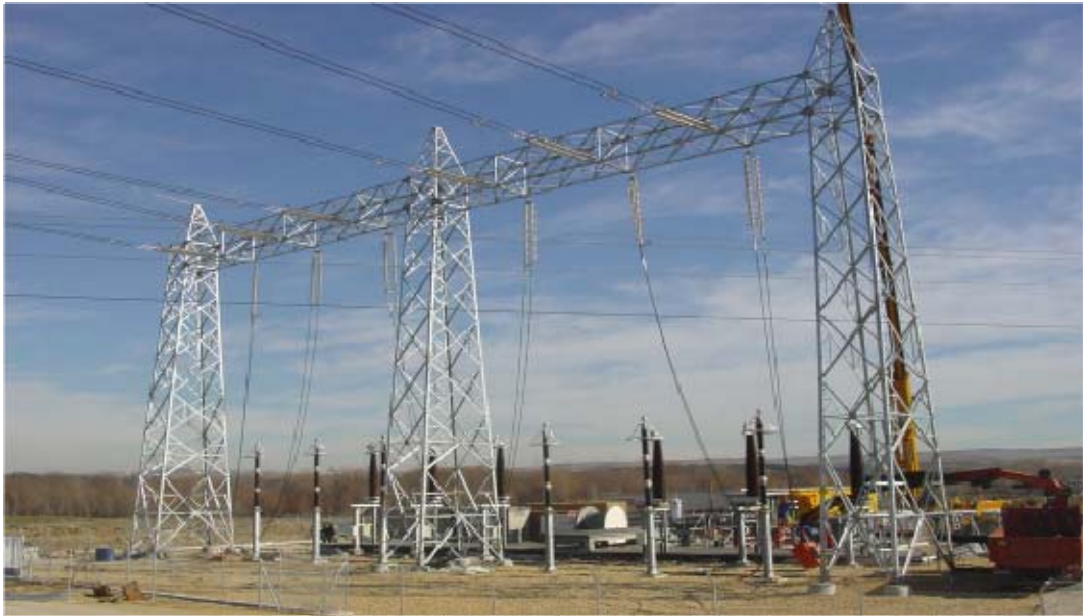
Figure 3.3: Typical Line/Cable Interface Compound
