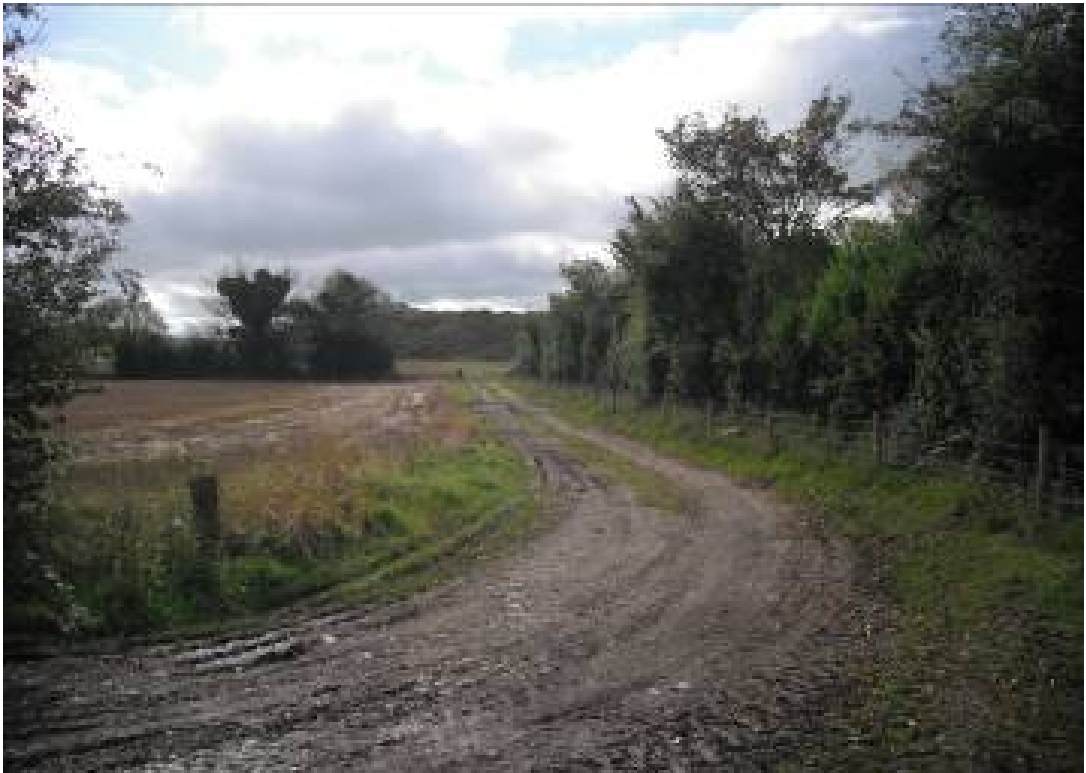
Figure 3.11: Existing Access to Proposed 400 kV Substation Site
