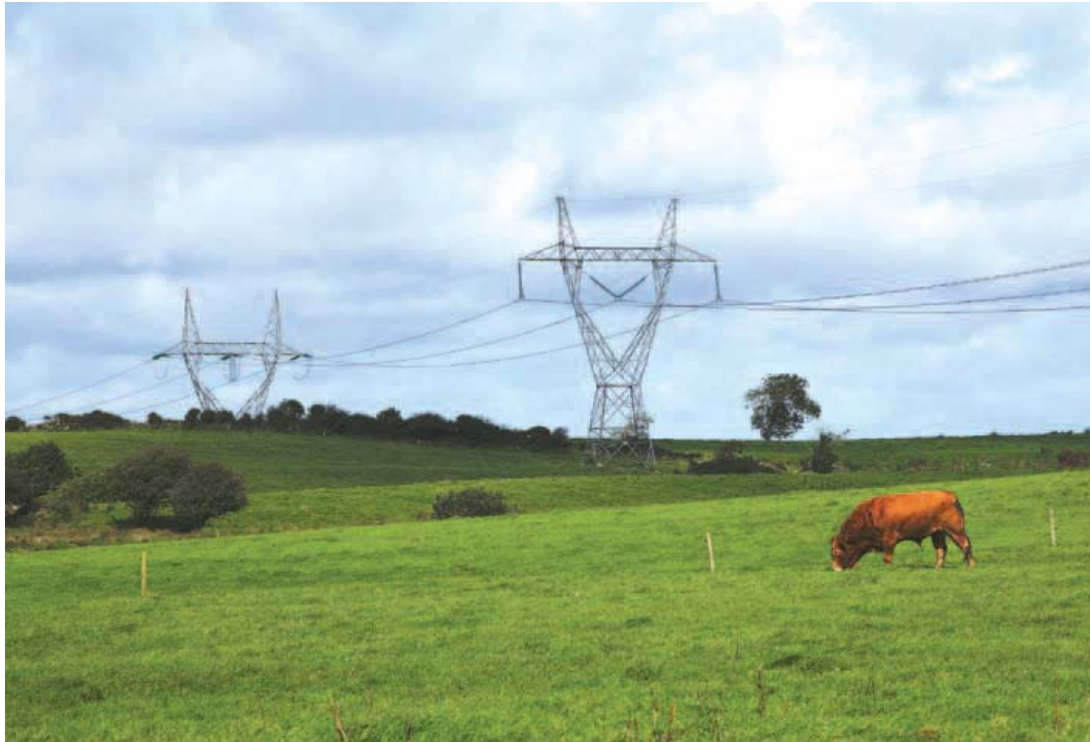
Figure 2.2: Photograph of 400 kV Single Circuit Intermediate Towers
